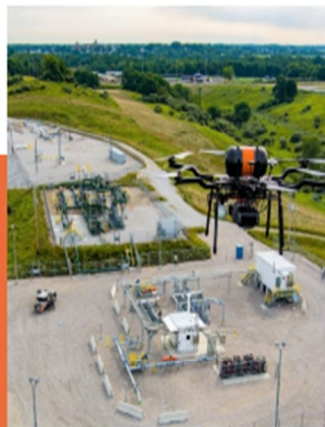
Pipeline inspection with Shell
