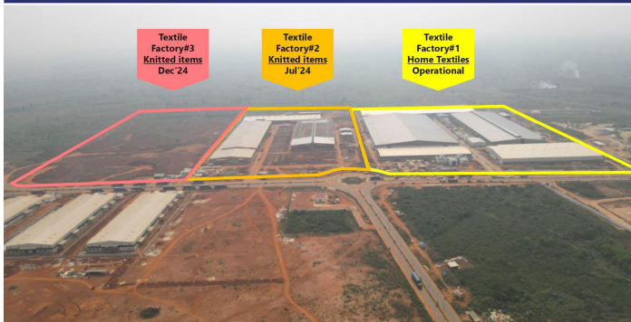
First 3 Vertically Integrated Textile Factories under construction
