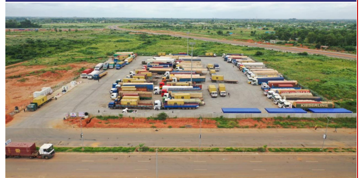
Inland Container Depot & Truck Parking
