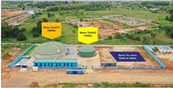
Borewells and Tanks to ensure 24x7 water supply
