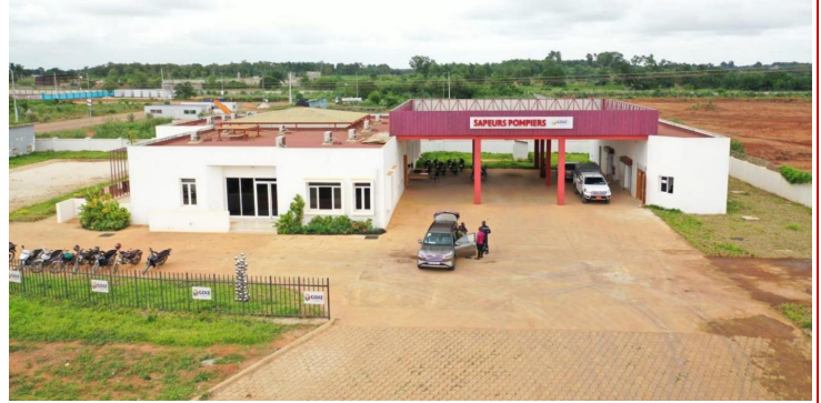
Dedicated Fire Station for the zone
