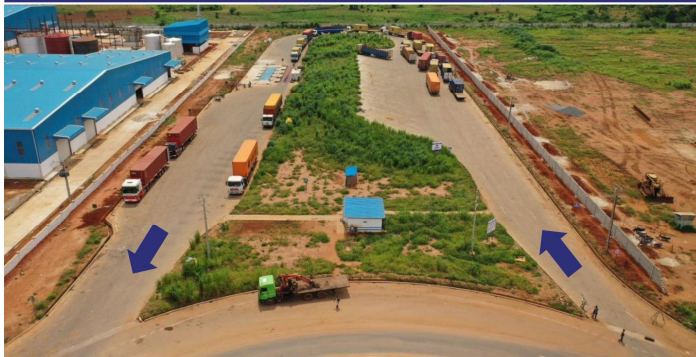
Weigh Bridge, Truck Parking & Driver Rest Area
