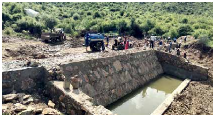
Work towards Ganga Wala Check dam is under progress
