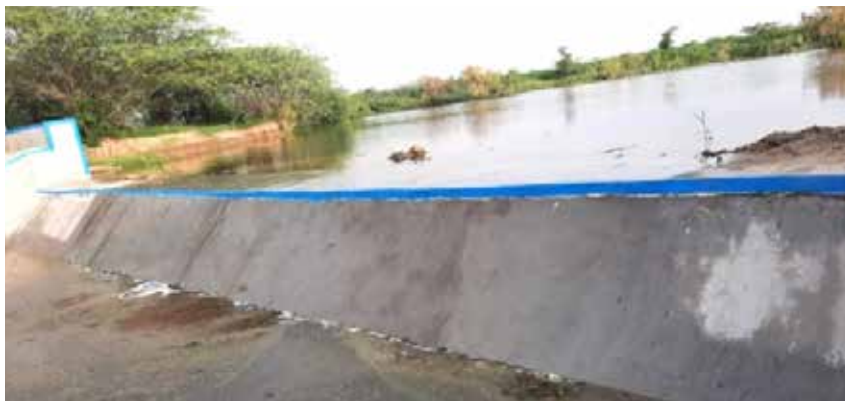
Completed Water Harvesting Structure at Pali, Rajasthan
