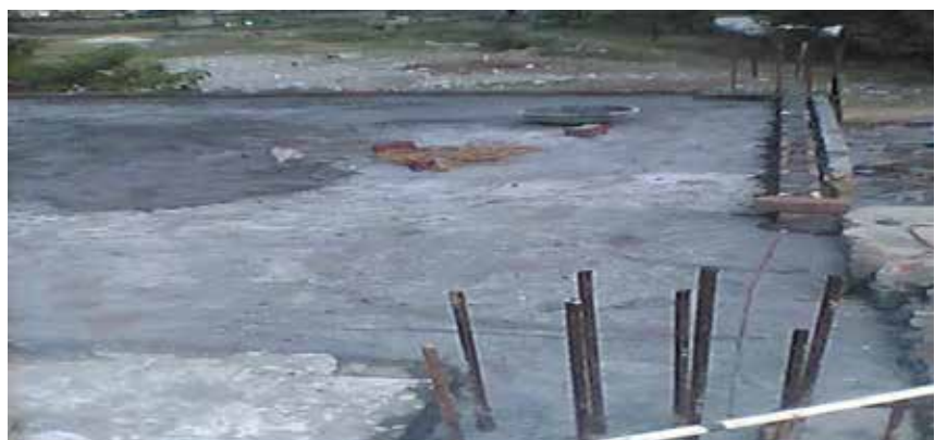
New Roof Casted
