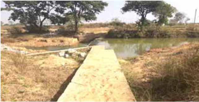
Gajam Wala Check dam at Ranchi, Jharkhand
