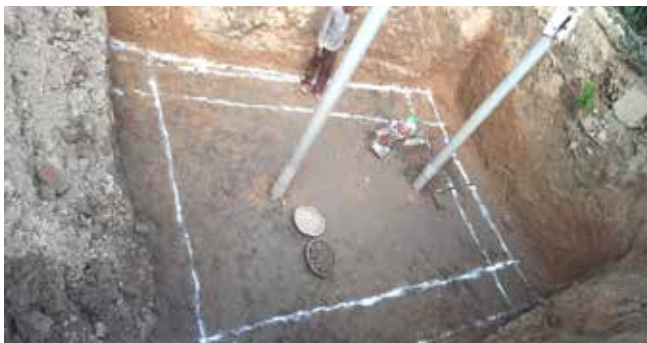
Excavation work in progress for establishment of rain water harvesting structure
