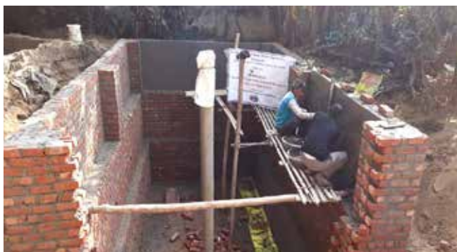
Construction work in progress for establishment of rain water harvesting structure
