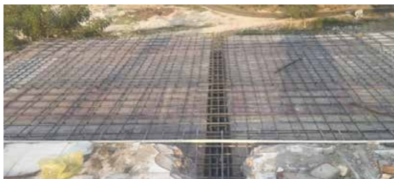
Iron Casting for RCC roof of a room in Junior Pathshala School in progress
