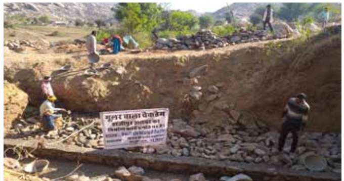
Foundation filling of Gular Wala Check Dam in progress
