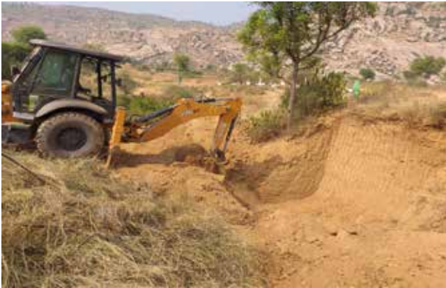
Excavation work taking place for Khali Kuan wala check dam
