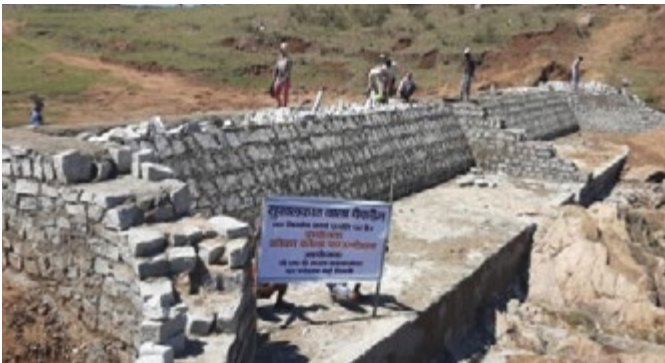
Construction work of Sukkhal Khatt Wala check dam in progress
