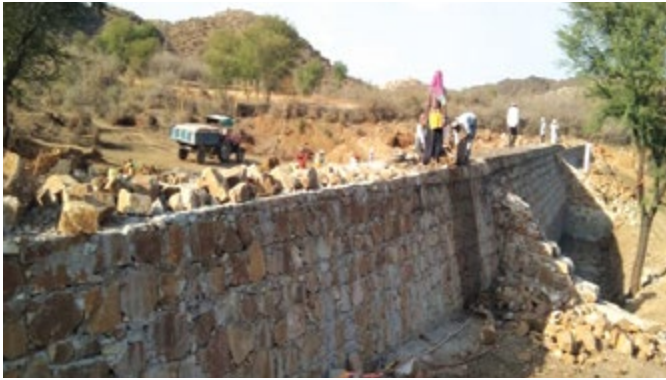
Construction work of Samra Wala check dam in progress
