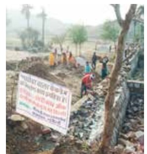
Work under progress of 'Pagthoda Wala' check dam in Jaipur, Rajasthan
