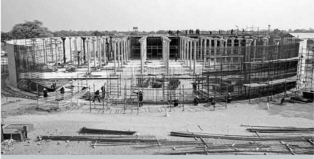
Photo of NamWater's 12,000m3 concrete reservoir under construction by a joint venture between B&K Civils and Rock Leigh Investments near the Ndama Water Treatment Plant on the Angolan border in Kavango Region. It was completed in 2018 to augment Rundu's water supply and will integrate with the AfDB's 'Water Sector Support Program' to Namibia (www.engineeringnews.co.za).
