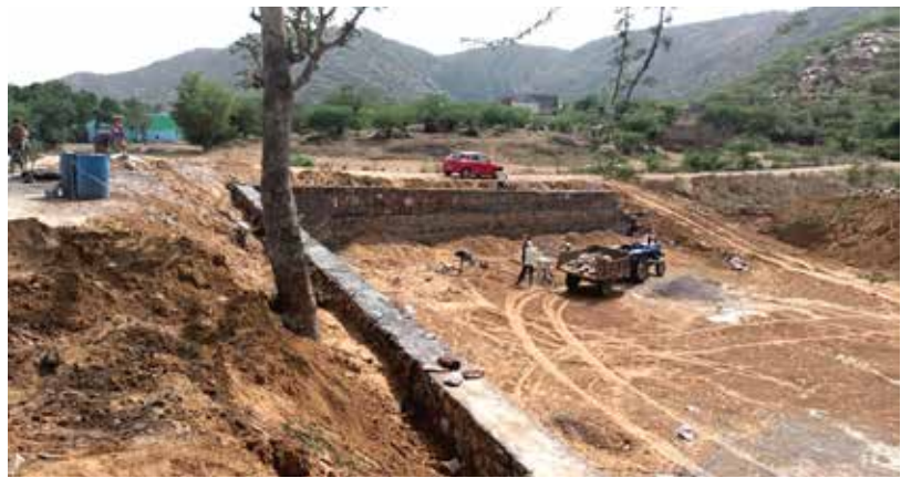
Gaushala Wala pond water harvesting structure work has been initiated
