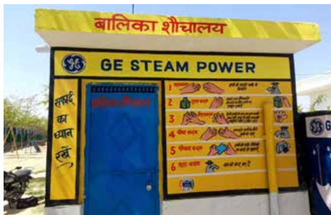
Toilet Block in one of the in Schools
