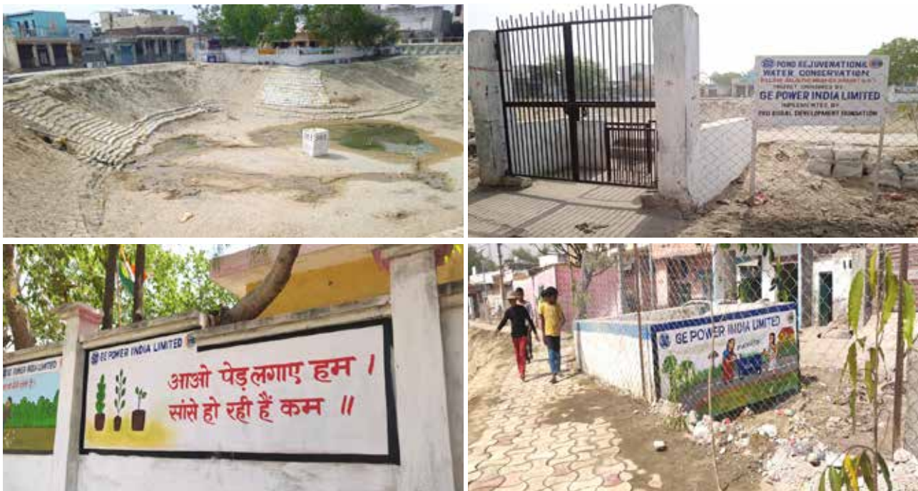
Work towards pond rejuvenation has been completed
