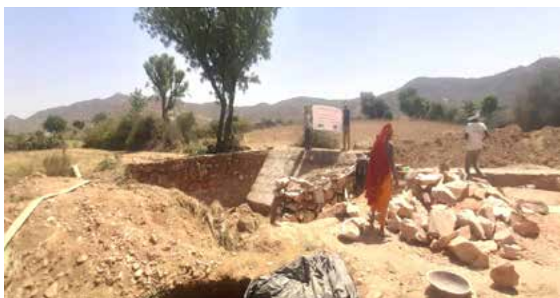
Lambibhat Wala water harvesting structure work has been initiated
