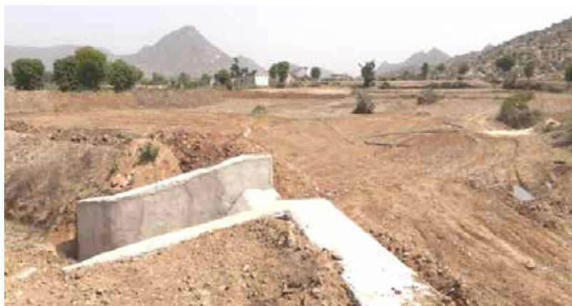
Waste weir has been completed and destillation work is under progress
