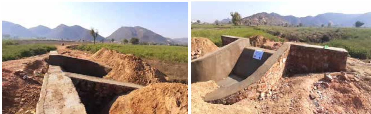
Establishment of Pyare Lal Wala water harvesting structures in progress
