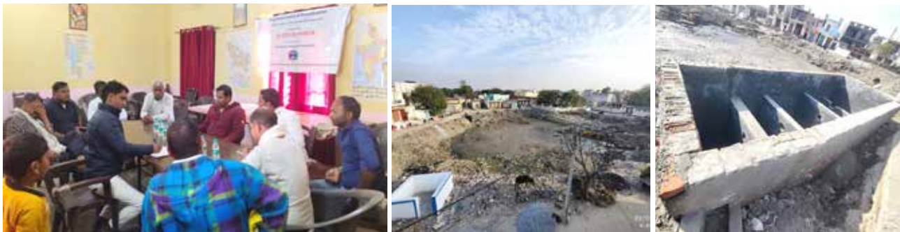
Rejuvenation of the existing pond in the Village Roza Jalalpur , Gautam Budh Nagar district in progress
