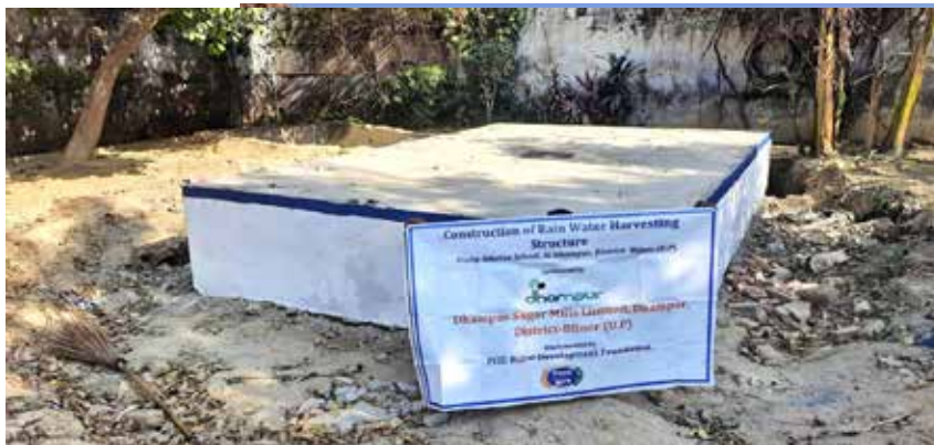
“Rain Water Harvesting” structure has been completed
