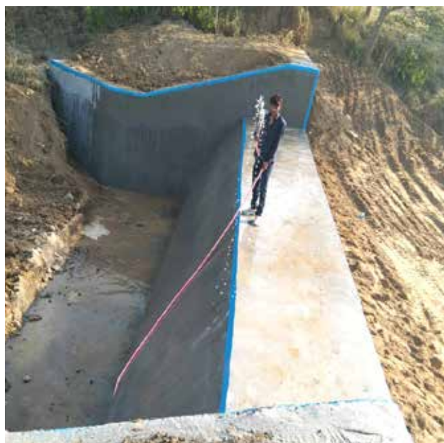
KundBawadi Wala Check Dam has been completed
