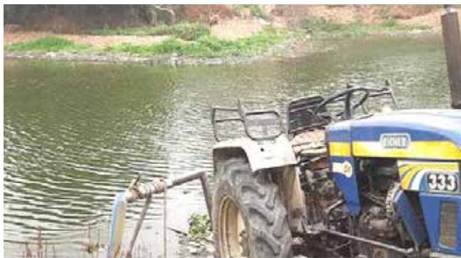
Dewatering work is on-going of Mohra Pond
