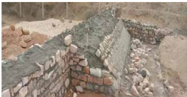
Dyalpura 3 & Dyalpura 4 wala Check dam establishment work under progress
