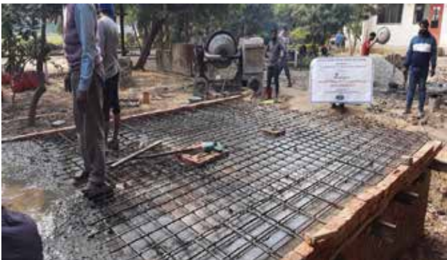
Two recharge shafts with depth of 45 m each are being established that will collect 7,347,000 litre of water
