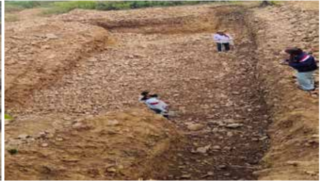
KundBawadiWala Check Dam
