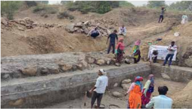
MandawariWala Check dam
