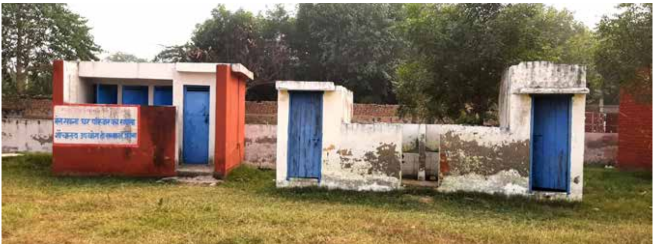
Existing toilet blocks in one of the proposed schools at Nuh, Haryana
