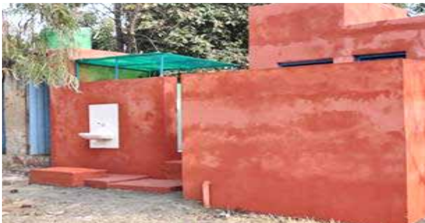
Two Blocks Refurbished in Mandothi School
