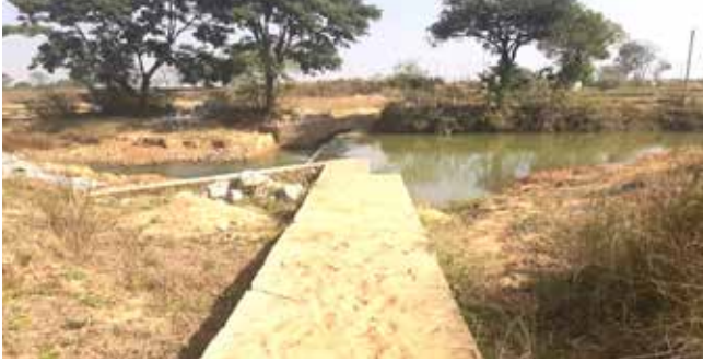
Gajam Wala Check dam at Ranchi, Jharkhand
