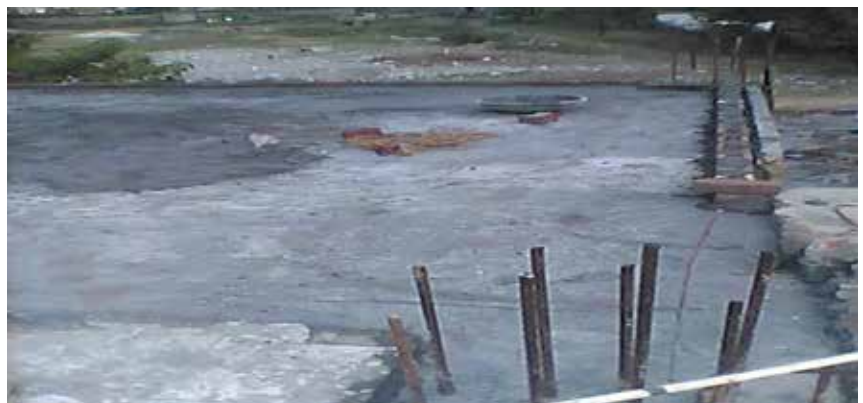
New Roof Casted
