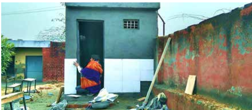
Construction under Progress in Rewasan School in Nuh
