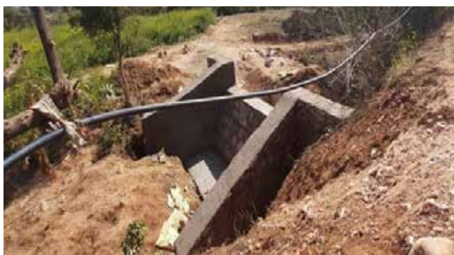
12 check dams have been constructed so far out of 51 structures
