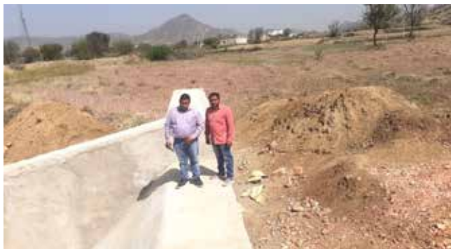
Waste weir has been completed and distillation work is under progress.
