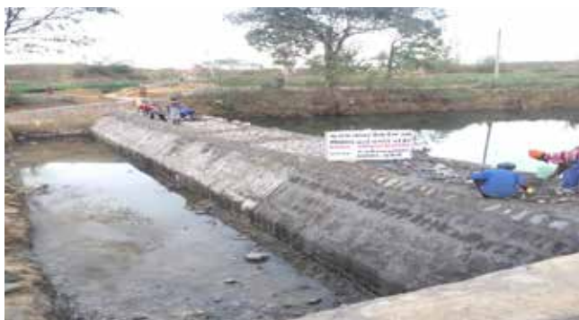
Ground water recharge, through construction of check dams
