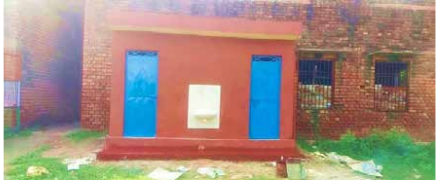
Newly constructed toilet block in Kulasi School
