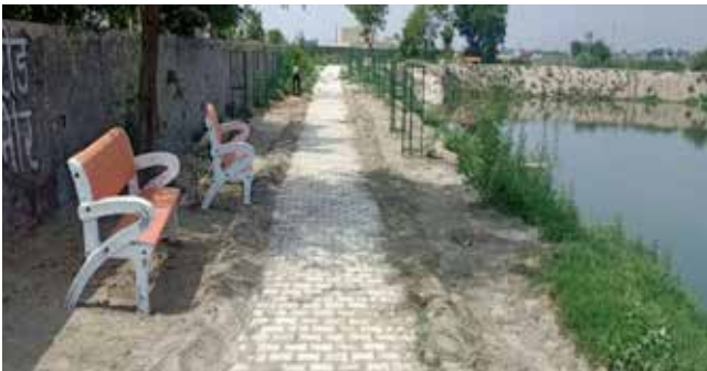
Pond beautification work has been completed
