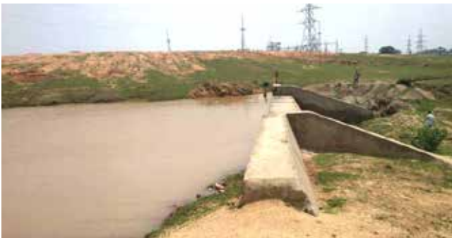
Five check dam has been completed out of seven
