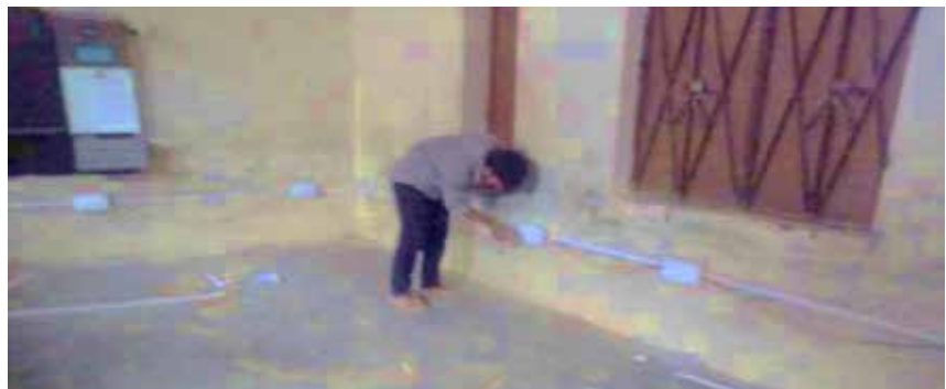
Electric Points Fitting in Naharpur School Being Done
