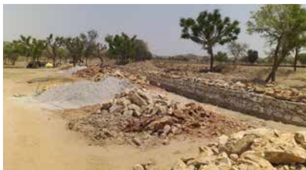
Construction work of ‘Sushil’ Check Dam in progress
